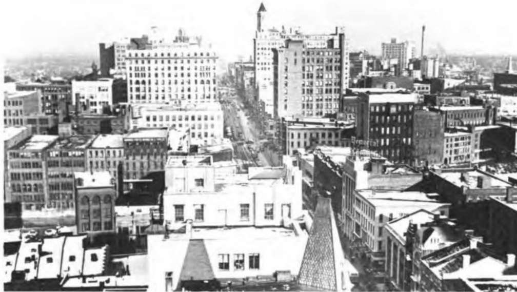
Twenty years later, with 95% of central downtown buildings heated with RG&E steam
