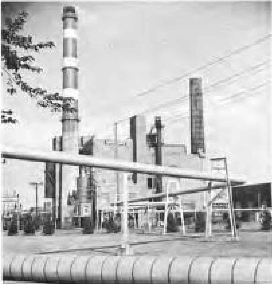
The Lincoln Park Building, better known as Station #9, where steam is generated for industrial use
