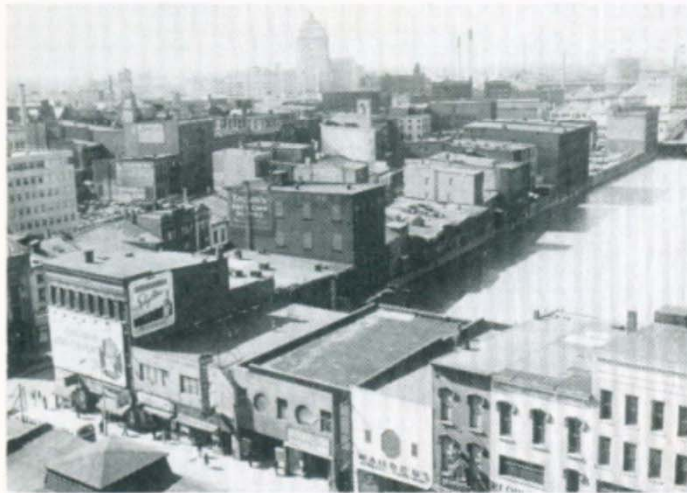
FIG. 1 — Old buildings on west side of Genesee River and on north side of Main St. crossing river, torn down in 1966-67 for urban development program.
