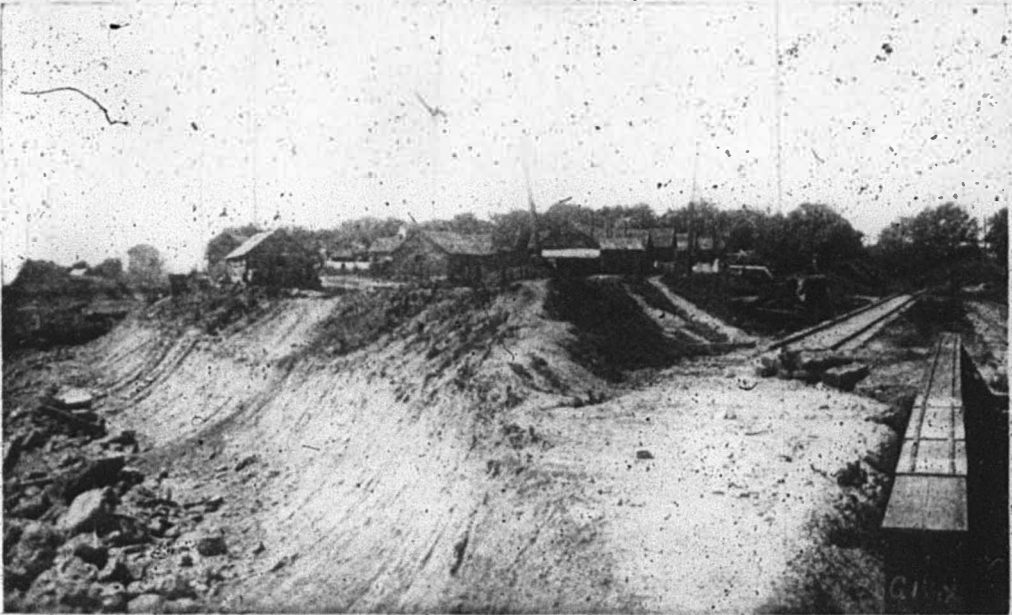
V IEW OF A LABOR CAMP ON THE BARGE CANAL: CANAL TO THE LEFT
