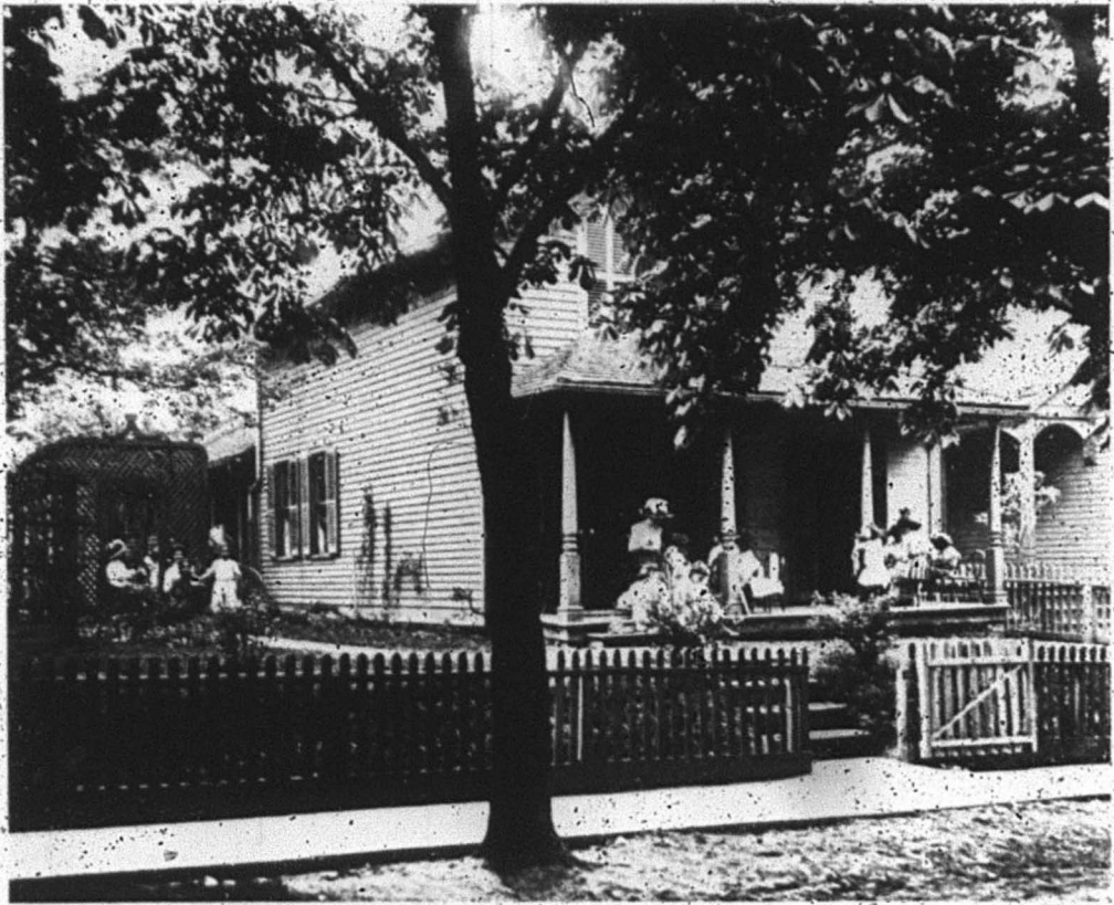
• The Housekeeping Center at 57 Lewis Street
