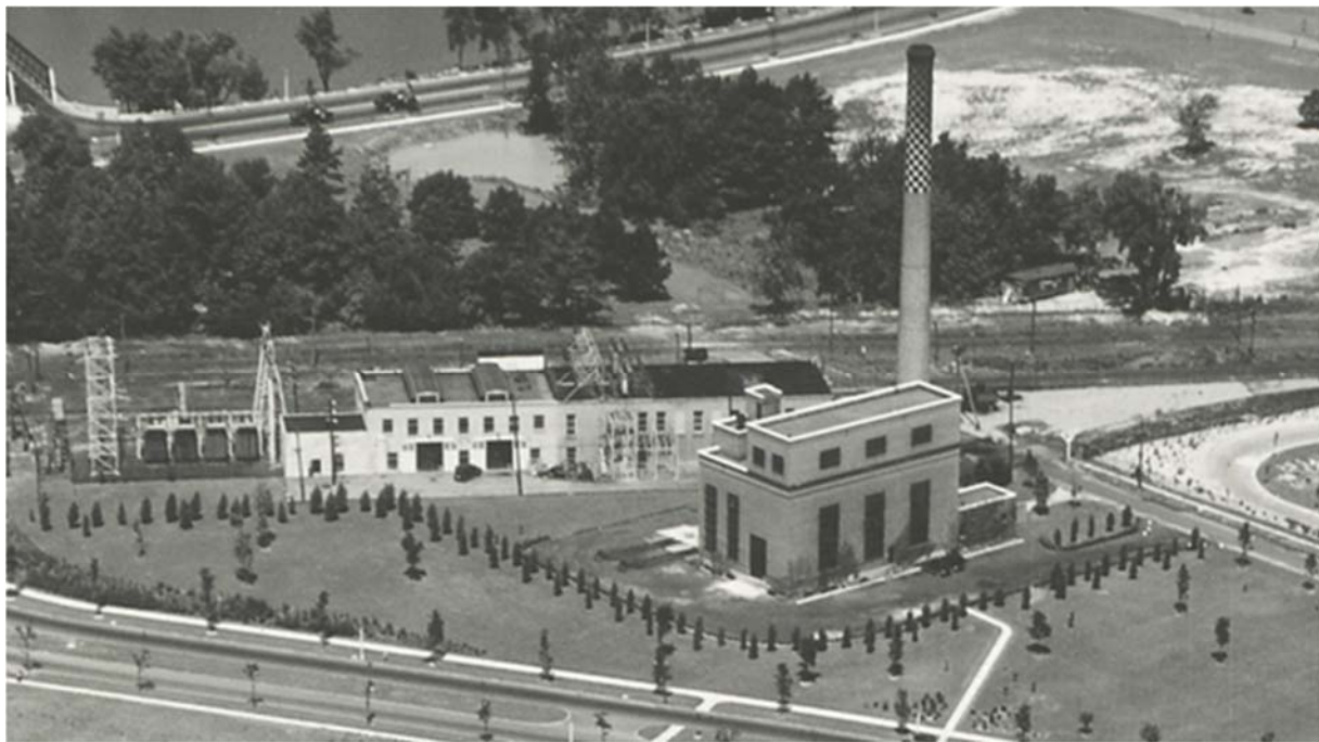
August 4, 1931 picture of the University of Rochester's Central Heating Plant adjacent to RG&E's Station 33.
