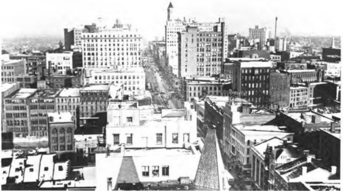
Twenty years later, with 95% of central downtown buildings heated with RG&E steam
