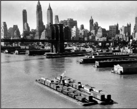
The Brooklyn Bridge, the East River, and the Downtown Skyline. Ewin Galloway. NARA 208-PP-62-22.
