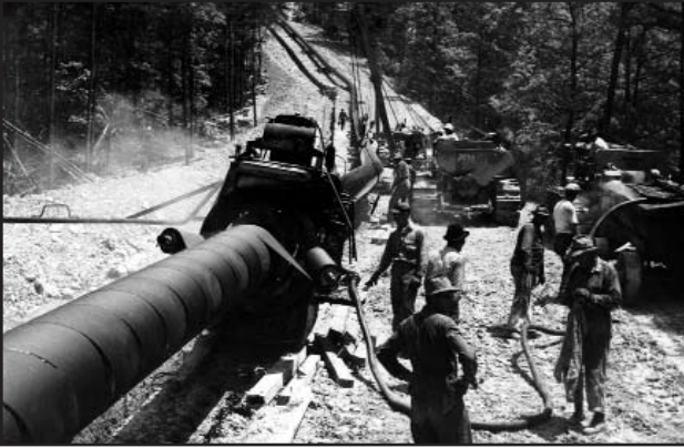
Machine wrapping pipe in felt. NARA 208-PRA-3-14-7126-44.
