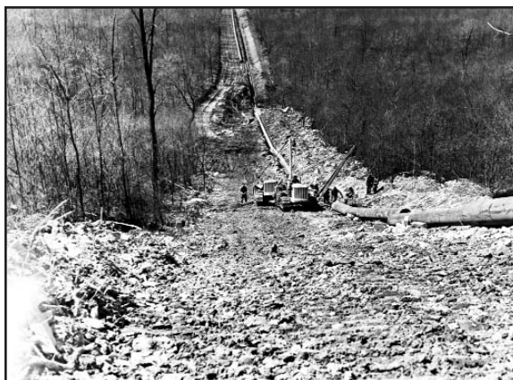
Swooping down the side of an Allegheny Ridge in western Pennsylvania, the "Big Inch" heads toward its other sections already nearing New York and Philadelphia. ACME. NARA 208-LU-37C-54.
