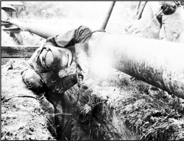
It's 99 in the shade, not counting the heat from the arc, as the welder joins the ends of two sections of pipe together. Pipeline welders work in pairs. World Wide Photos. NARA 208-LU-37C-36.
