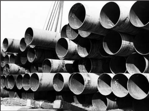
Pennsylvania section of the war emergency 24-inch pipeline carrying oil from the Texas fields to eastern refineries, completed in July 1943. Pipe stacked along the railroad tracks. John Vachon. NARA 208-LU-37C-50.
