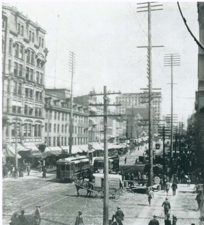
Rochester's Main Street in the early 1880's when telephone poles and their crossarms towered over the street.
