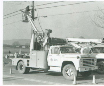
In the far left photo, a crew installs cable along the shores of Sylvan Lake in Dutchess County; near left, a Highland lineman fastens cable to a strand of wire in the 1970's.
