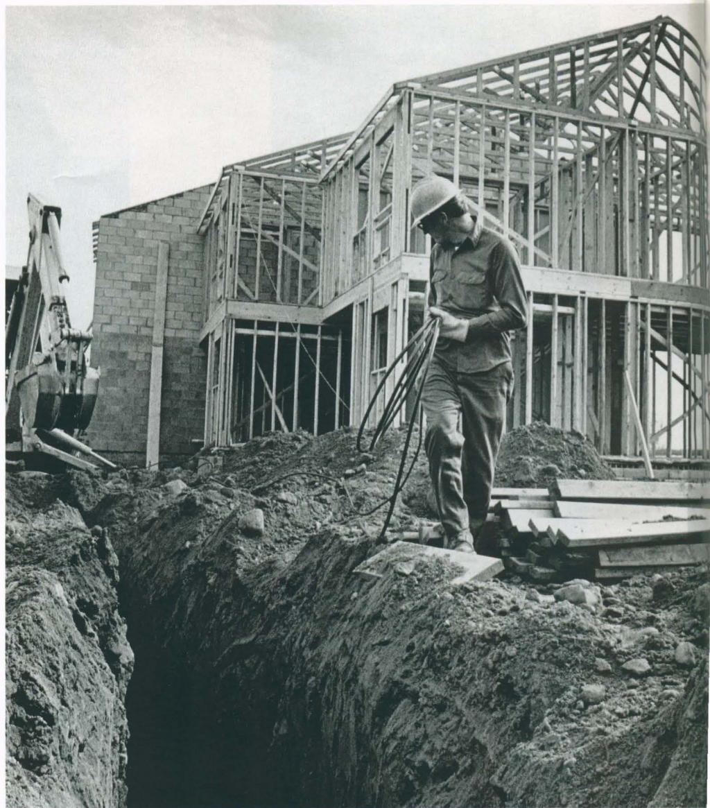
A lineman prepares to bury cable in one of the many housing developments that sprang up throughout the Rochester area in the 1960's and 70's.
