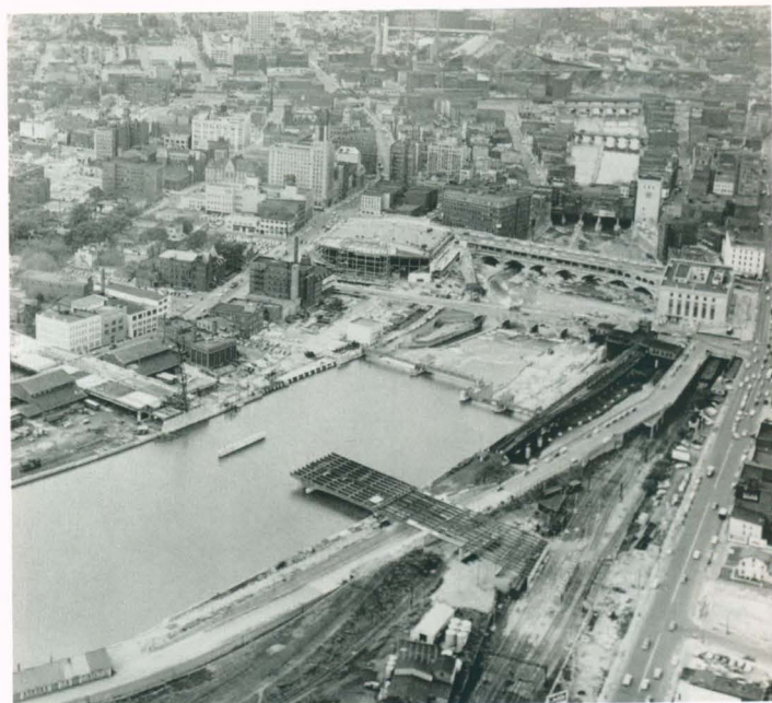
A view of downtown Rochester in the early 1950's when the Troup-Howell bridge, in foreground, and the Community War Memorial, upper center, were both under construction.
