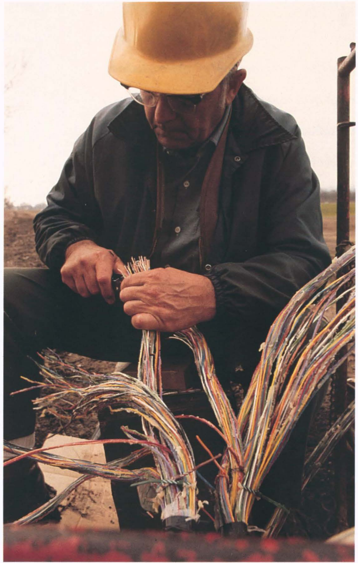
First stripping the ends of the wires, cable splicer John Maier works on a subscriber cable at the site of a new housing development in the early 1970's.
