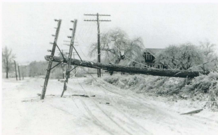
One of the hundreds of poles downed in the 1929 ice storm.
