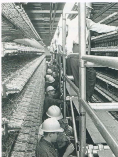
In the early hours of January 17, 1965, workers await the signal to disconnect the company's first dial equipment at Stone Street and activate a new crossbar office; above, the "tombstone" for the old Rotary dial office.
