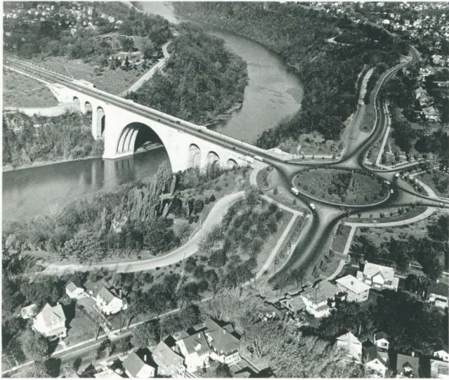
The Veterans Memorial Bridge under construction in 1931 and, below, after its completion, with the St. Paul Street traffic circle at right.
