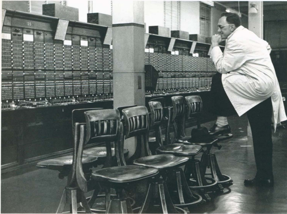
On the night in 1961 when the last manual office in Rochester was cut to dial service, the company's traffic manager, John Banks, has a final look at the deserted switchboard, which just hours before was alive with people and voices.
