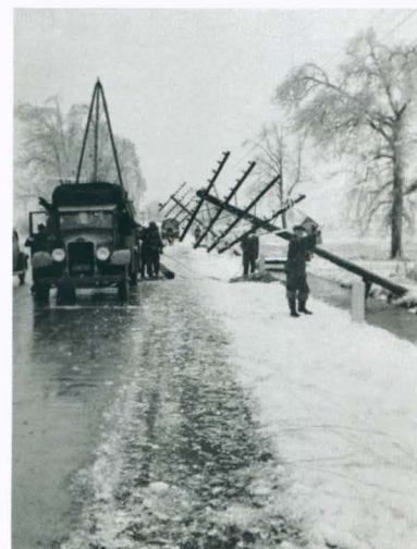
The aftermath of the 1936 ice storm; the area outside Rochester was especially hard hit.
