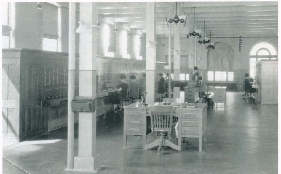
The switchboard room on the second floor; initially, 26 positions were equipped for operators.
