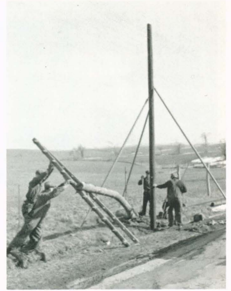
A line crew removes an old pole after installing a new one.
