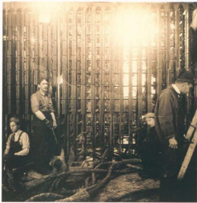
Rewiring the Stone Street frame after the 1908 fire.
