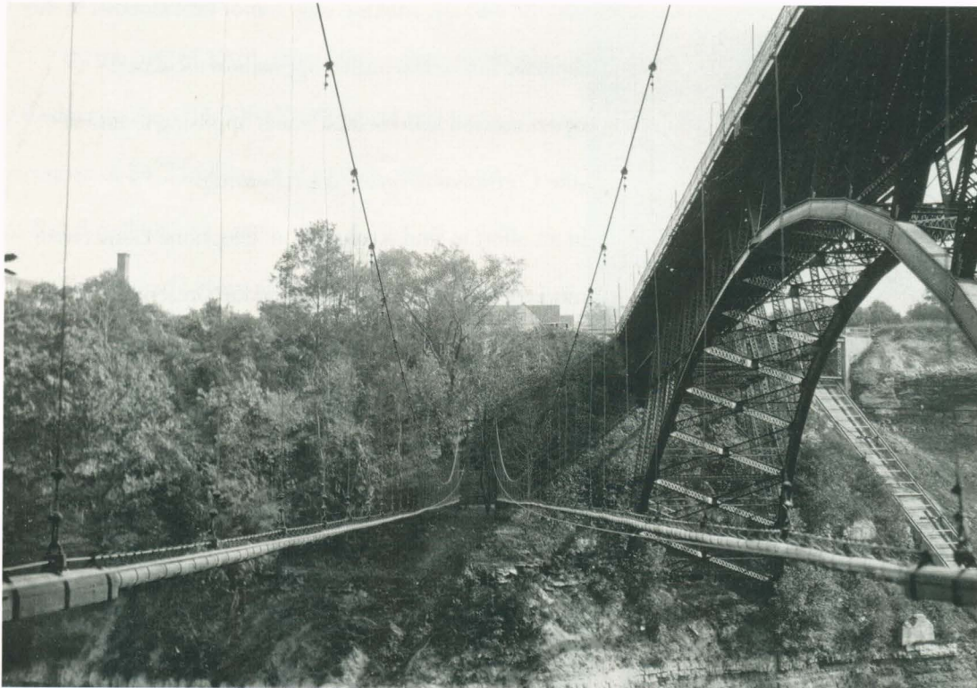
Stretching 462 feet across the Genesee River near the Driving Park bridge, these 900-pair cables were the longest aerial cable span in the world when installed in 1923 and 1924.
