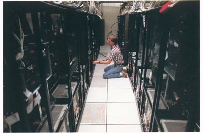
A Rotelcom installer, Jaye Lang, working on the installation of a Rolm switch at the University of Rochester. Completed in 1987, Rochester Telephone served as the general contractor for the project, which was the largest ever undertaken by Rotelcom.
