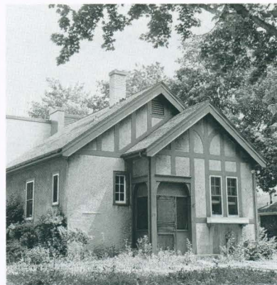
Just 33 years to the day after it was opened in 1932, this manual office in the village of Honeoye Falls was abandoned in 1965, and later razed, after the community was cut over to dial service.
