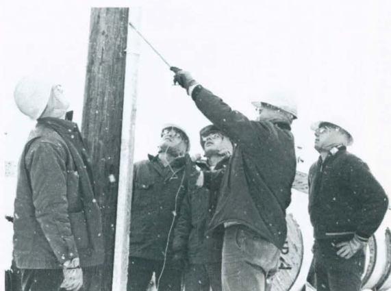
New linemen are shown how to check a pole for electricity before climbing.
