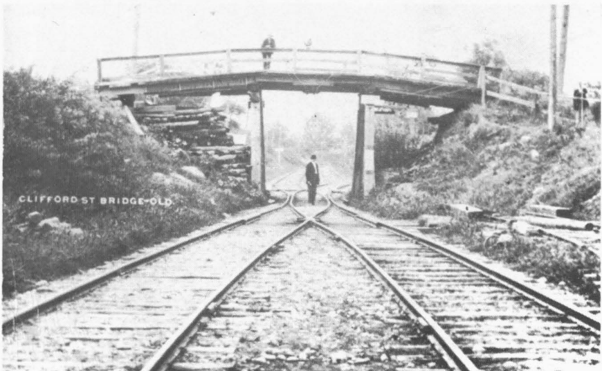
Old bridge on Clifford Ave., now is Empire Blvd., gauntlet track under bridge.
