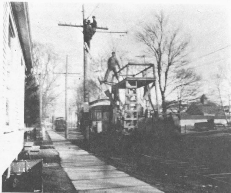
Line repair car and trolley on Beach Ave. at Charlotte. Note wooden side walk. 1900.
