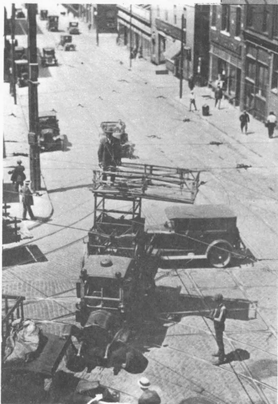
Looking down Andrews from St. Paul, July, 1925. Man on raised platform is repairing trolley wire. Rings bell on roof when in a hurry.
