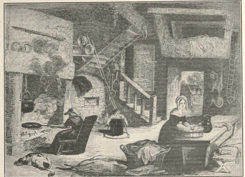
An 18th Century kitchen. Note the fireplace and at its right the round Dutch brick oven, opening into the fireplace at the side.
