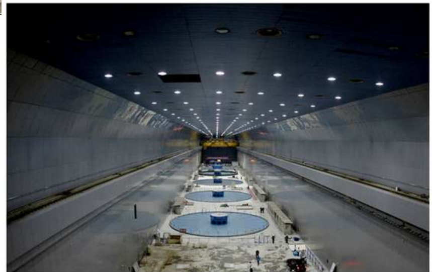
Photo taken on July 4, 2012 shows the interior scene of the Three Gorges' underground power station in Yichang, Central China's Hubei province. [Photo/Asianewsphoto]
