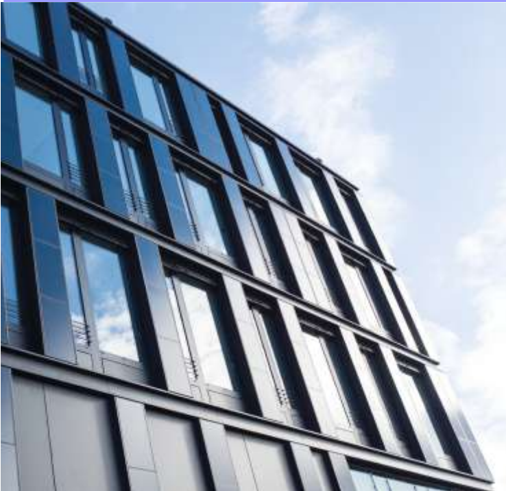
The ZSW institute's building in Stuttgart-Vaihingen has a façade with CIGS panels.
