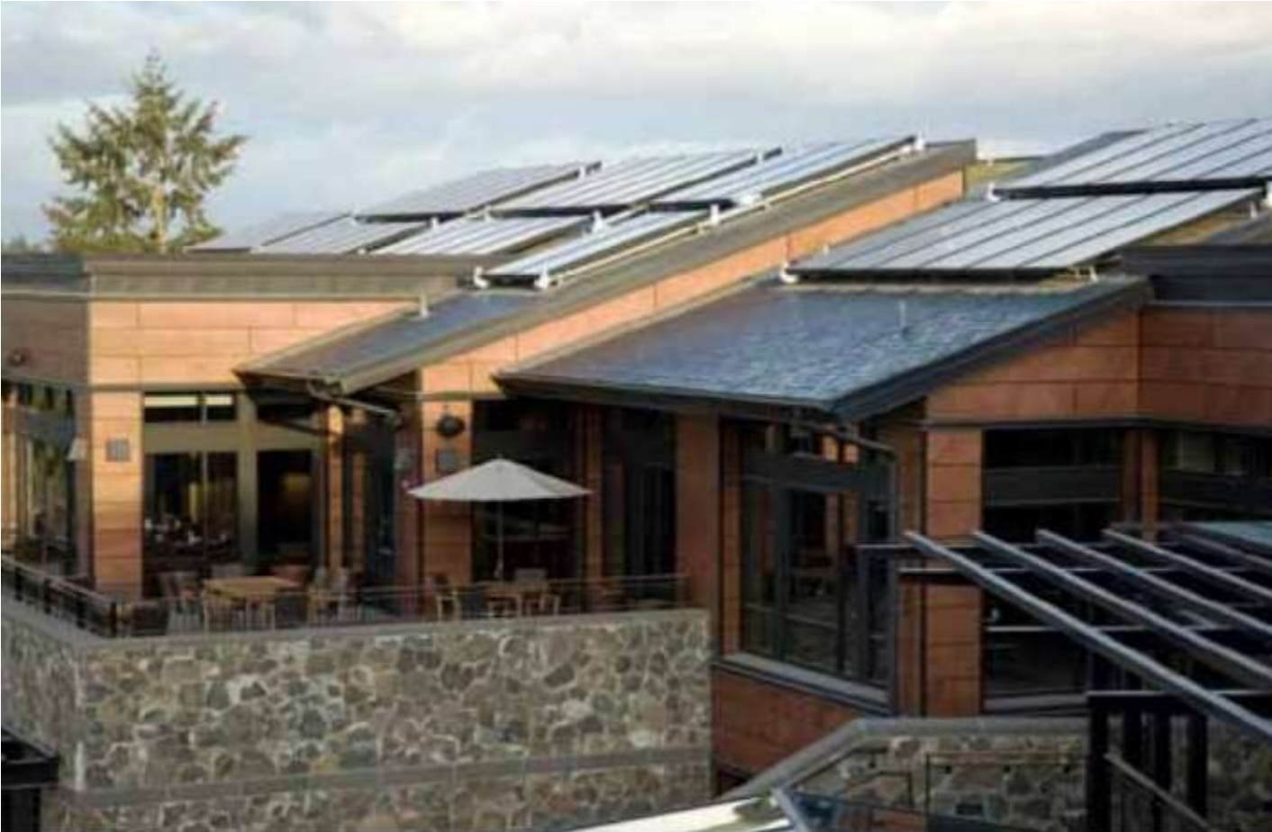
Solar thermal installation at the Allison Inn, Oregon
