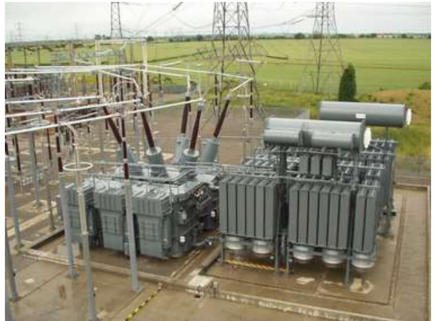
Cooled power transformer on national e-grid
